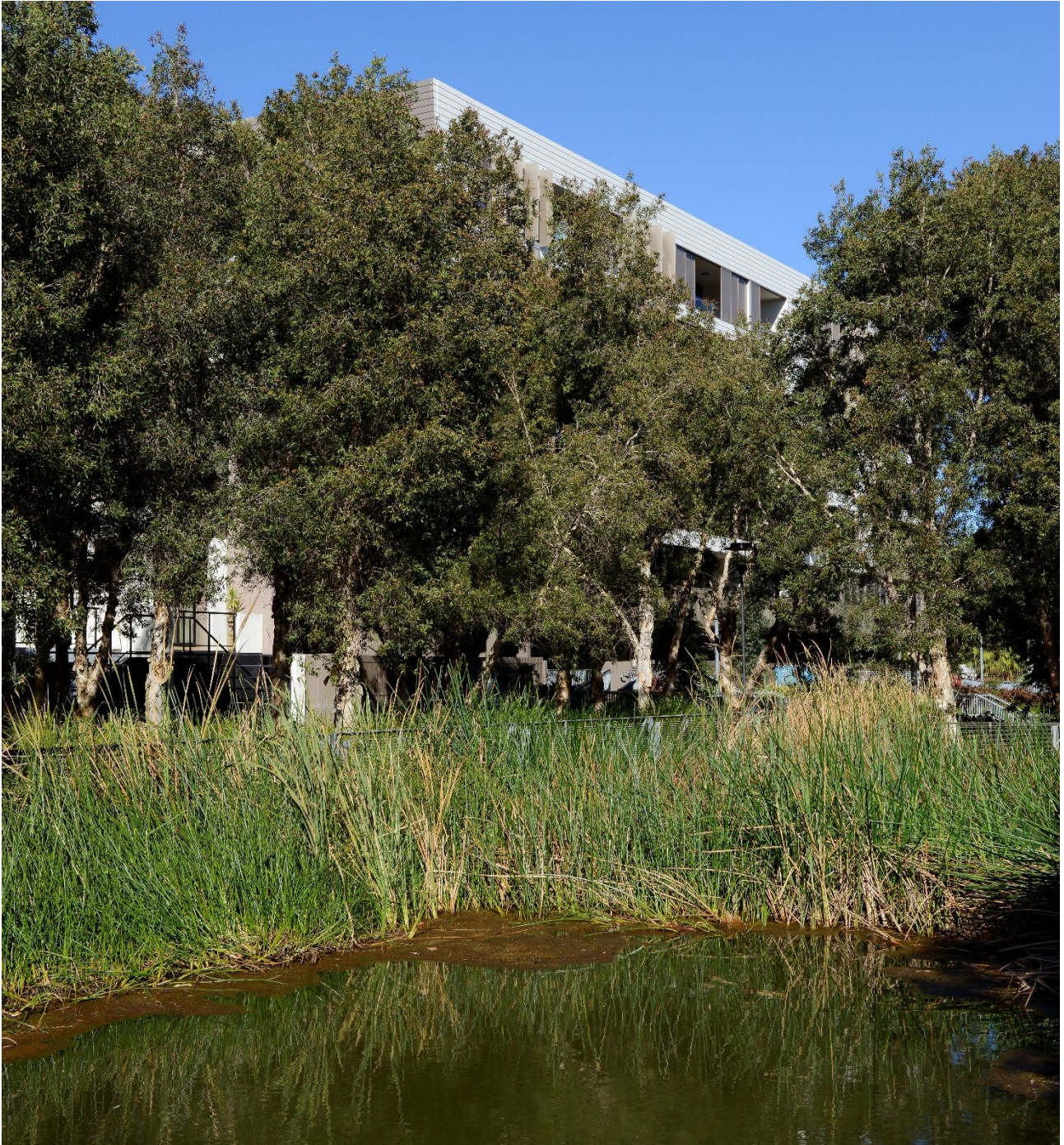
Image 4. Wetland reconstruction and drainage on Joynton Avenue. Image: Adam Hollingworth/City of Sydney
